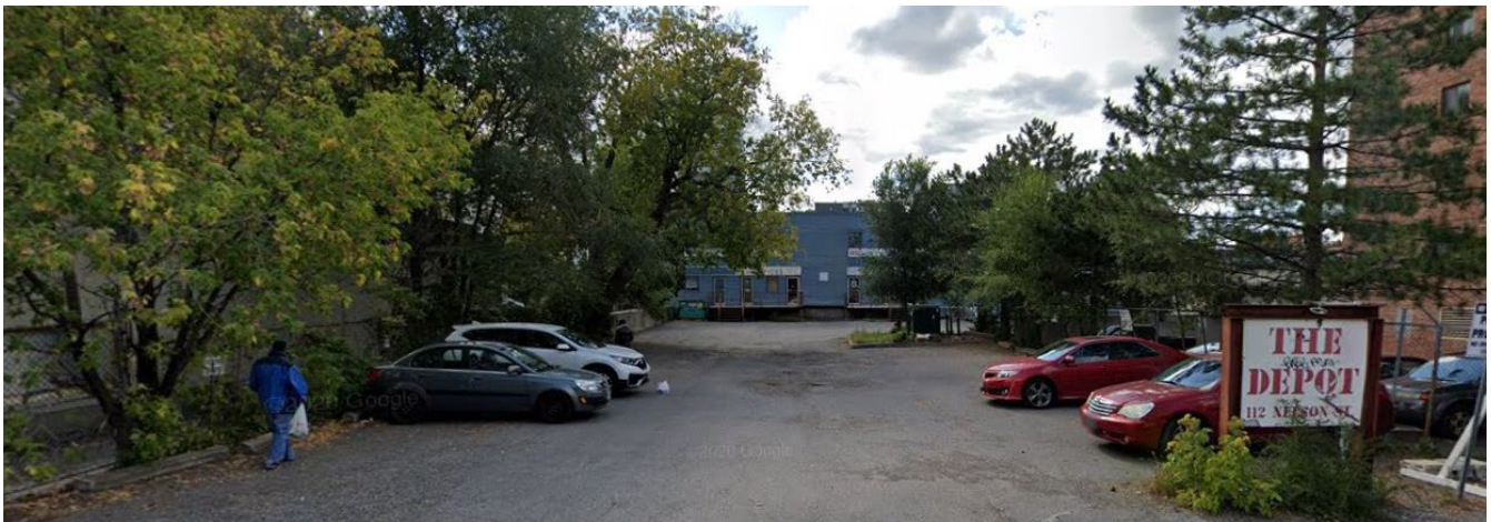
Figure 2: Existing building on the subject property, view from Nelson Street.
