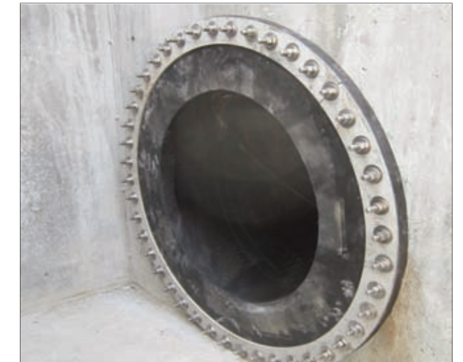
Upstream Flanged CheckMate®
