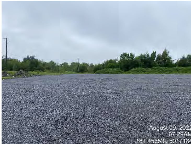
Photo 2 - View of ground improvement area.
