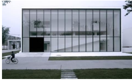
Glass curtain wall for the main building access facade (Cluster D)
