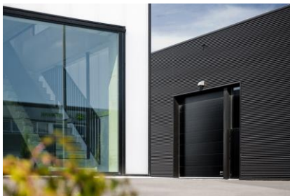
Big glass openings for specific locations, like the offices and lunchrooms
