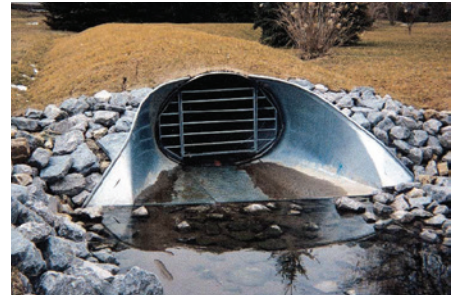
CSP END SECTION WITH FUNCTIONAL GRATE
