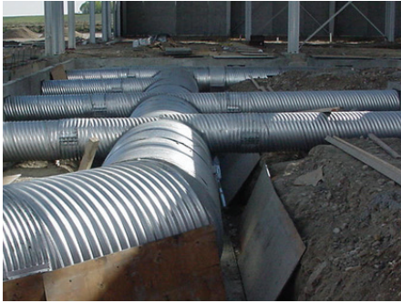
CSP CAN BE FABRICATED TO SUIT A MULTITUDE OF CONFIGURATIONS
