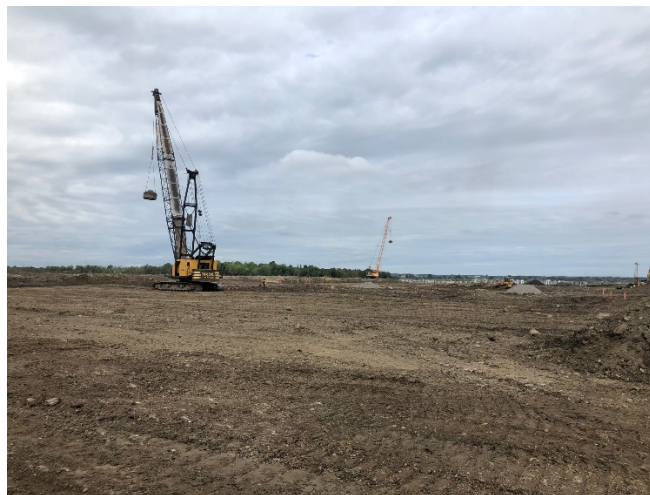
Figure 1. Dynamic Compaction Rig – Ottawa, ON
