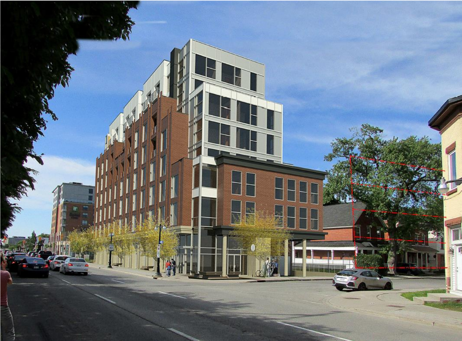
View looking north from the intersection of King Edward Avenue and Clarence Street.
