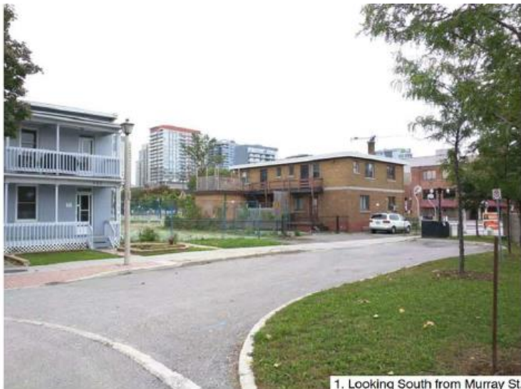
1. Looking South from Murray St.
