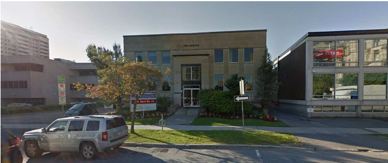
Figure 2: 100 Argyle Street, frontage and building
