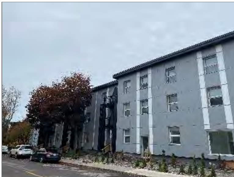
Photo 2 – Site Building (south elevation).
