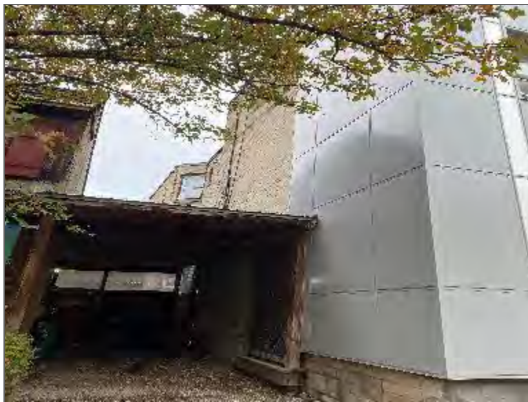
Photo 4 – Site Building (west elevation).
