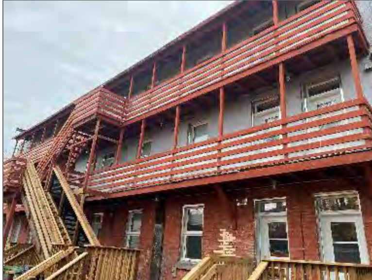
Photo 1 – Site Building (partial north elevation).
