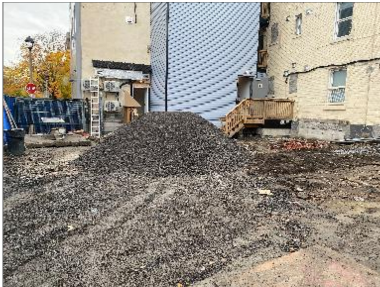
Photo 6 – Former parking lot (currently being graded for future development) on the northeast portion of the Phase One Property.
