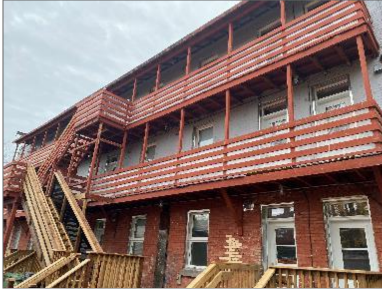
Photo 1 – Site Building A (partial north elevation).
