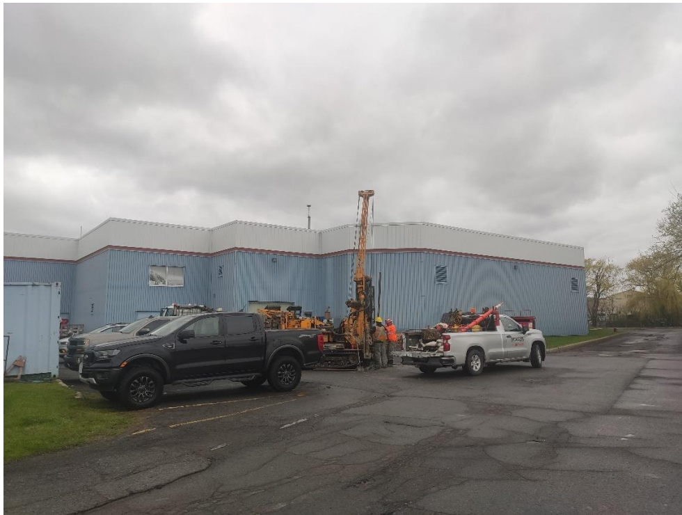
Figure 2 – Drilling with CME-55LC during May 5, 2021 mobilization
