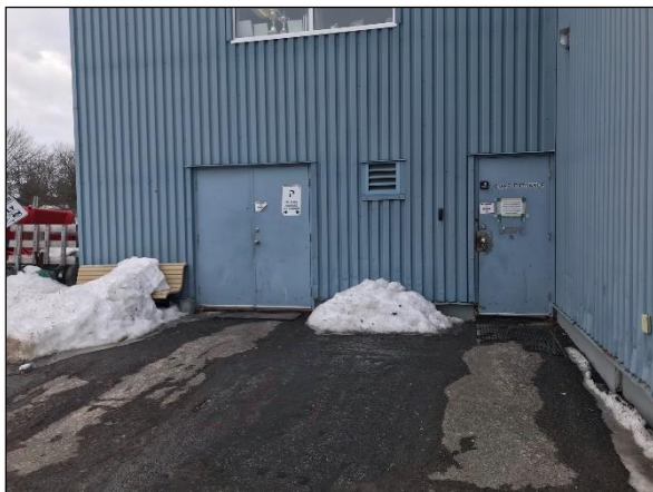
Back entrance (northeast side) of arena
