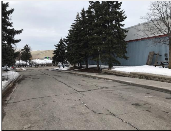
Front of building – facing northwest
