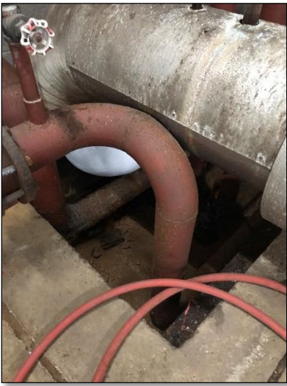
Plant room – trench for chilling system
