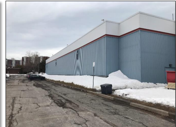
Parking lot – southeast side of the building
