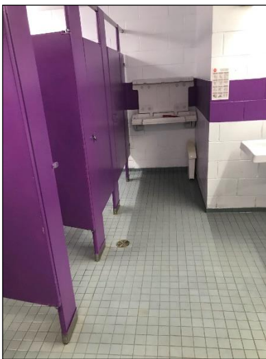
Main floor washroom
