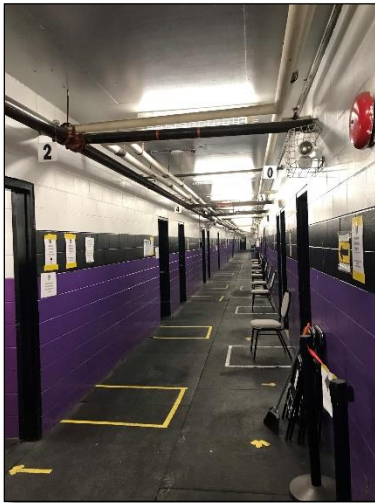
Low floor – change room access
