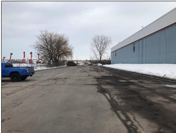
Parking lot – northwest side of building
