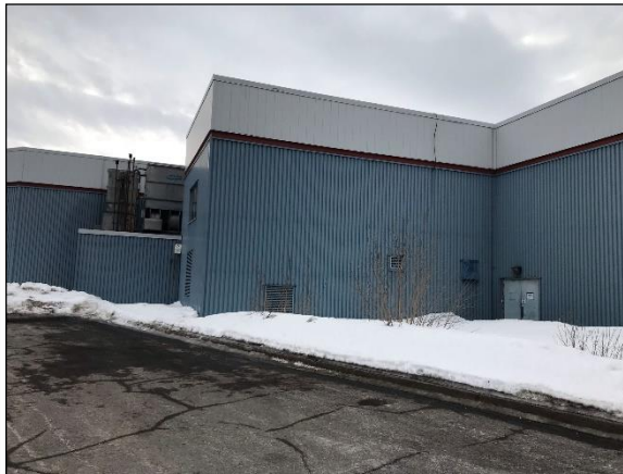
North corner of building – condensers on rooftop for chilling system
