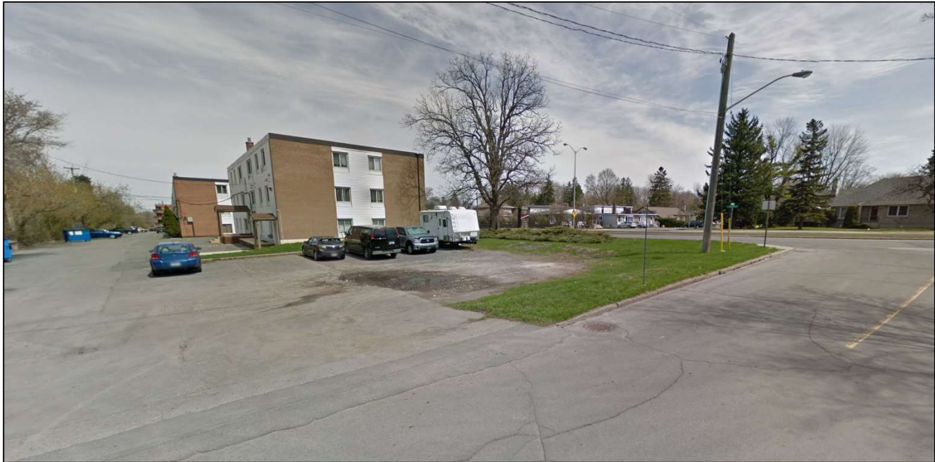
Exhibit E-3: Photograph of site of Proposed Development at the Subject Property (May 2014) from Bromley Avenue
