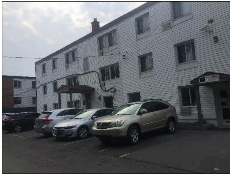
Photo 3 – Site Building C (northwest elevation).
