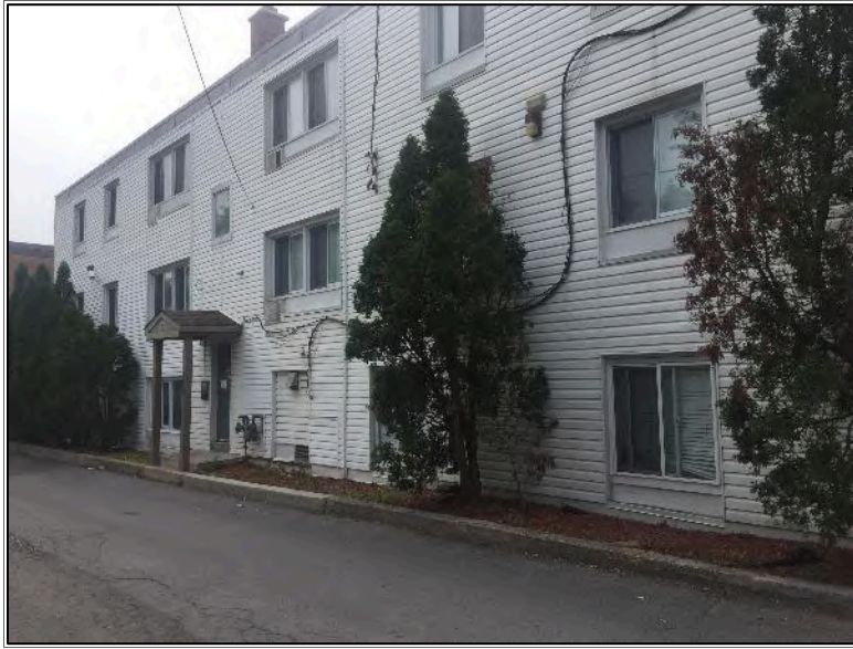
Photo 1 – Site Building A (northwest elevation).
