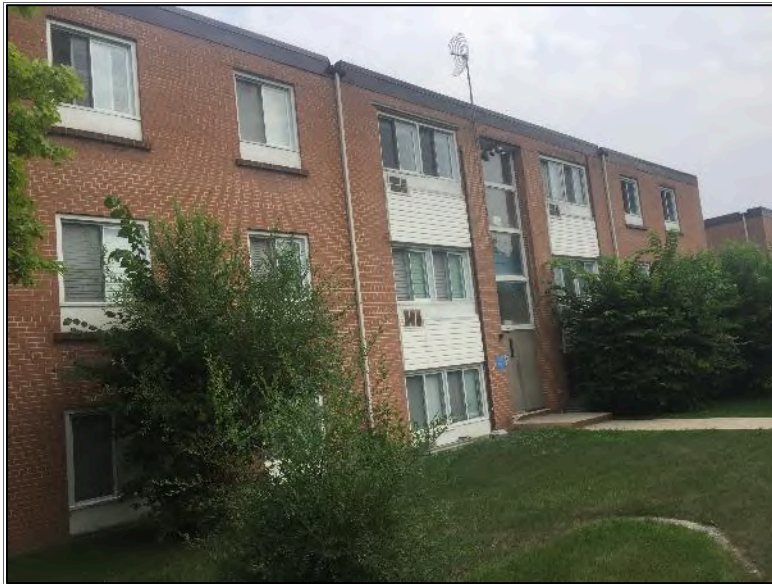
Photo 2 – Site Building B (southeast elevation).
