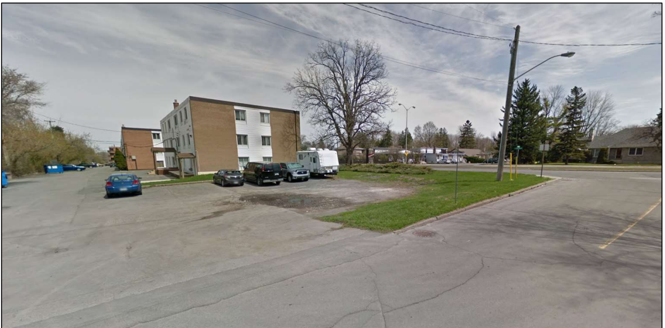
Exhibit E-3: Photograph of Area of Redevelopment of Subject Property (May 2014) from Bromley Avenue
