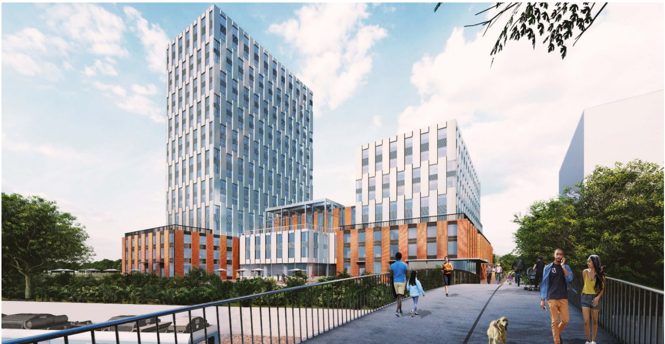
Figure 9 View from future Laurel Active Transportation Bridge looking east.
