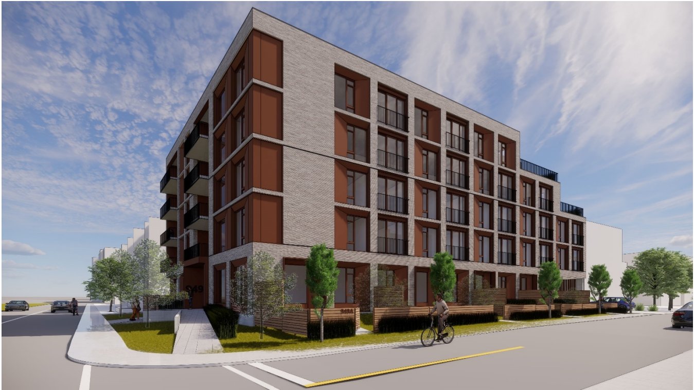
Figure 10: Looking northeast towards the proposed development
