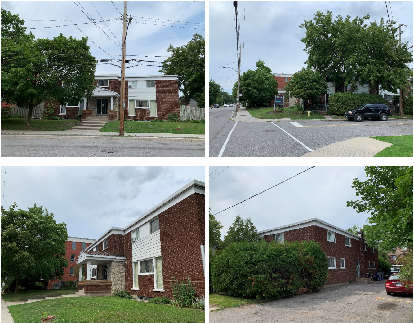
Figure 2: Top Left, looking west towards the subject site; Top Right, looking north towards the subject site from Ontario Street; Bottom Left, looking along the front property line of the subject site; Bottom Right, looking northwest towards the rear of the subject site
