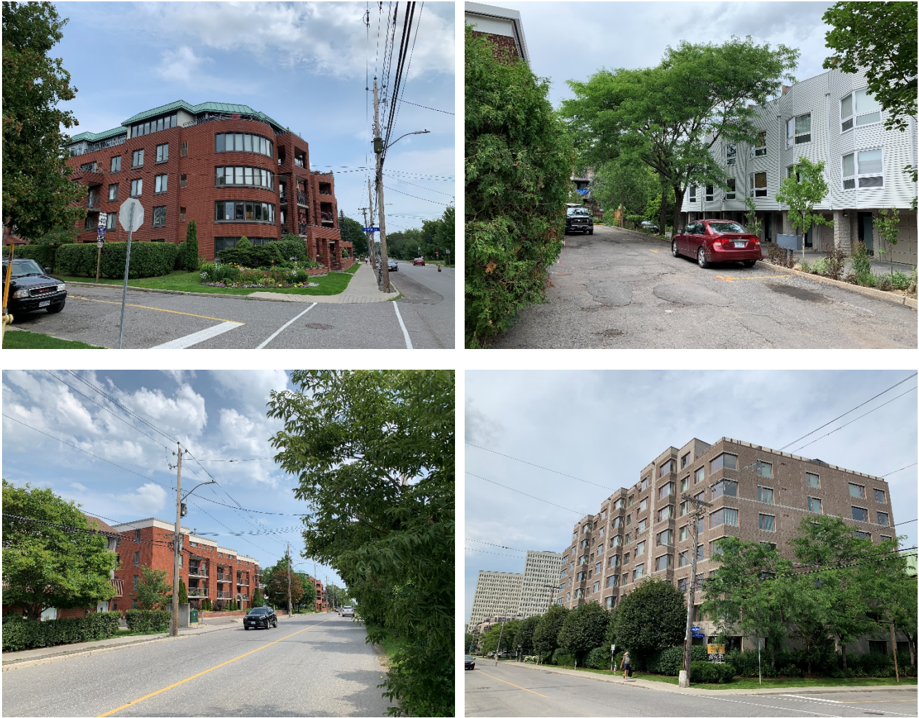
Figure 4: Top Left, looking south across Ontario Street to five-storey property; Top Right, looking towards properties abutting the subject site to the south; Bottom Left; looking south along River Road to four-storey property to the north; Bottom Right, Eight-storey apartment located one block north of the subject site
