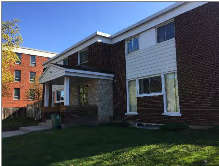
Photo 4 – Site Building (west elevation).
