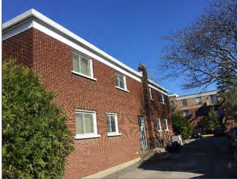
Photo 3 – Site Building (east elevation).
