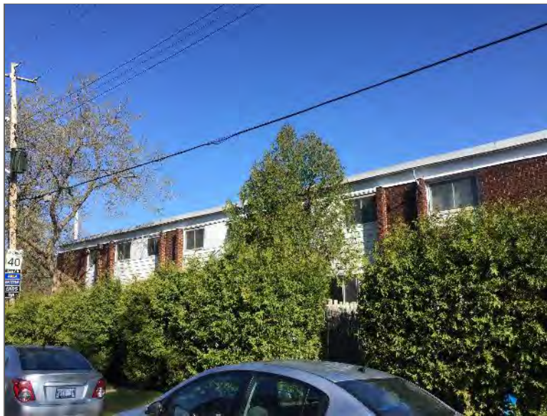
Photo 2 – Site Building (south elevation).
