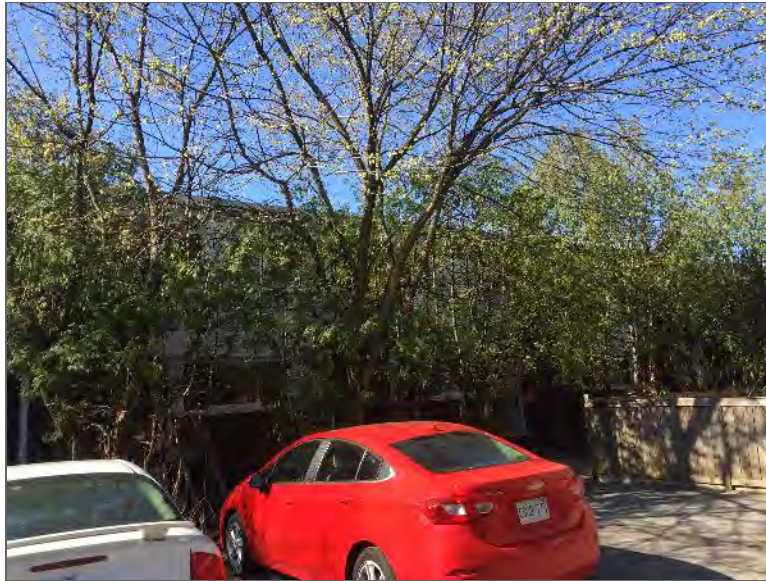
Photo 1 – Site Building (north elevation).
