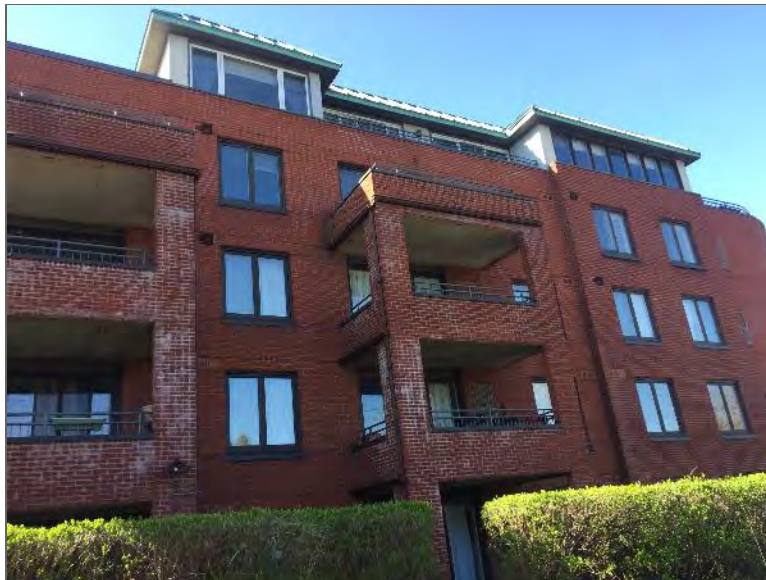
Photo 6 – Property located south of the Phase One Property.
