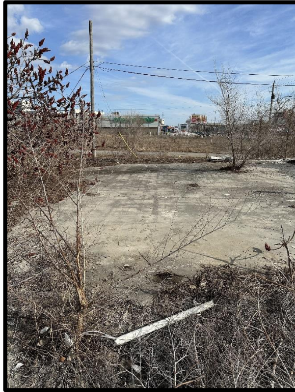
Photograph 1: View of the concrete slab on the Phase I-ESA Property, facing north.
