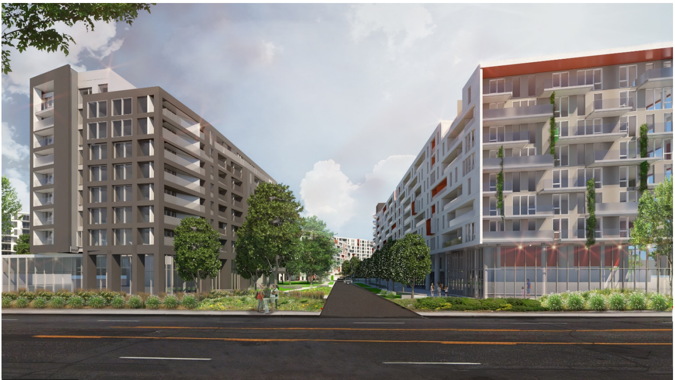
Figure 10: Looking north to site from Merivale Road
