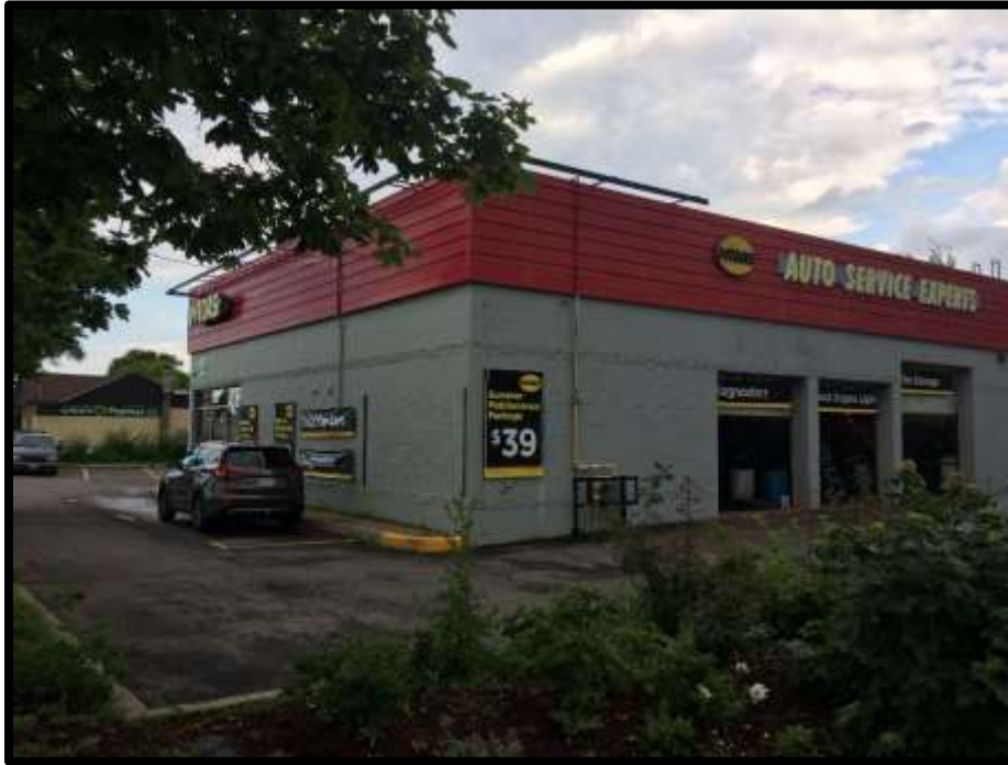
Photograph 7: Existing Midas building along Baseline Road
