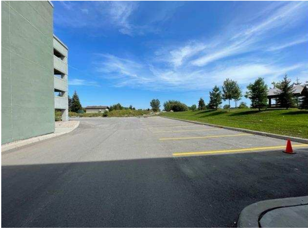
Photograph 1: View of the southern half of the Phase I ESA Property, looking east.
