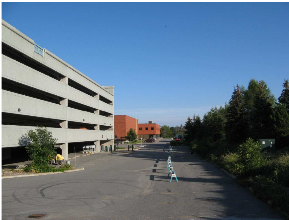
Photo 1 – Location of proposed apartment building adjacent to existing parking structure. View looking north towards Terry Fox Drive with conifer plantings on a grassed berm to the left. Berm will be removed
