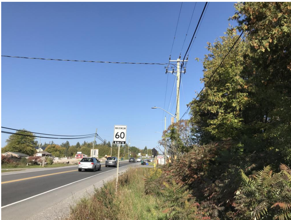
Photo 4: View of powerlines running along Carp Road.
