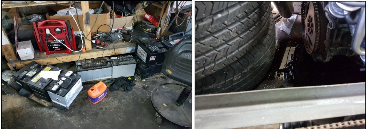
Photograph 12 and 13: View of the battery storage (left), note pooling liquid underneath the motor in the Vic's Automotive unit (April 9, 2018).
