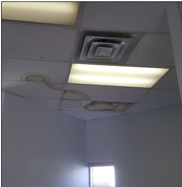
Photograph 14 and 15: View of water damage observed in the Hertz tenant unit. Water infiltration due to roof sealant issues.
