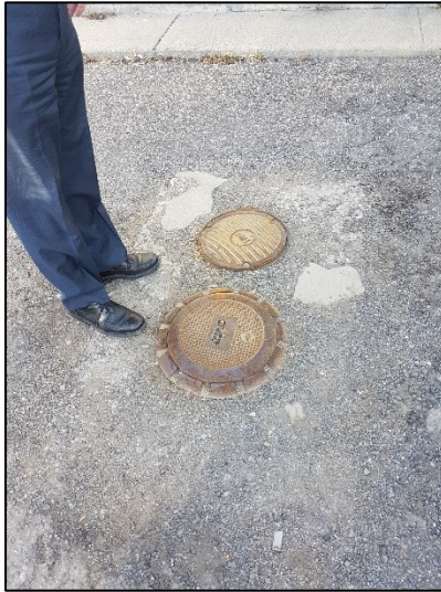
Photograph 5: View of unidentified access ports observed adjacent to the south elevation of 2600 Bank Street (Site) (April 9, 2018)
