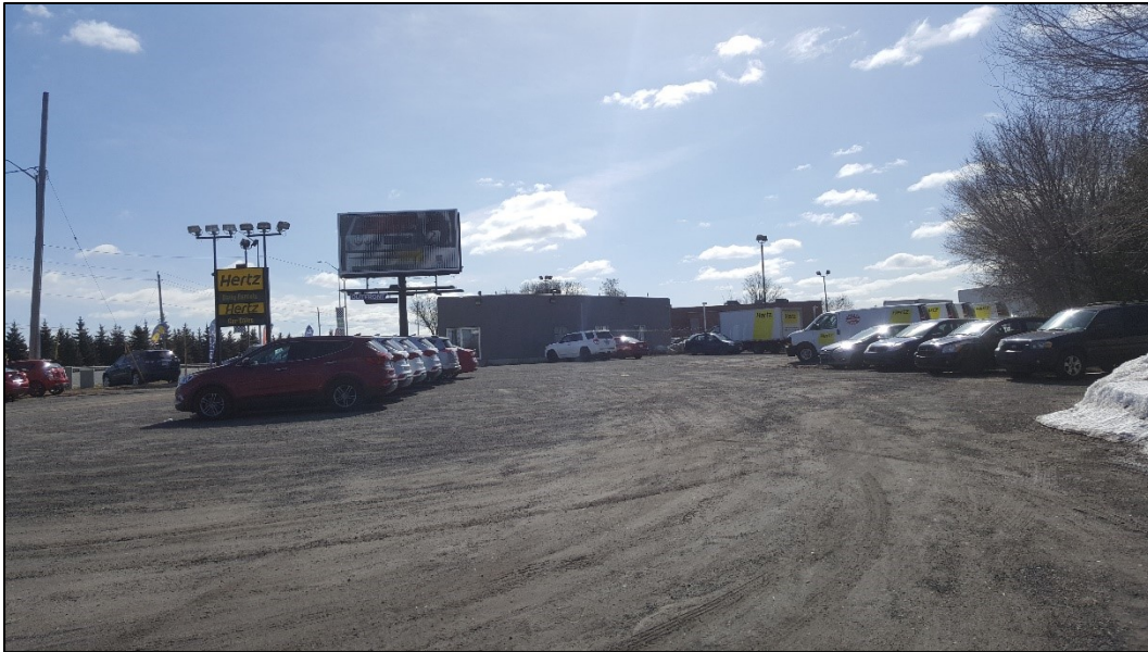
Photograph 3: View of western elevation of Site building (2600 Bank) and the side gravel parking area, looking east (April 9, 2018)
