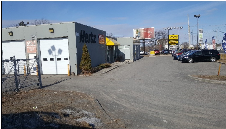
Photograph 1: View of northeast corner of the Site building, facing north (April 9, 2018)
