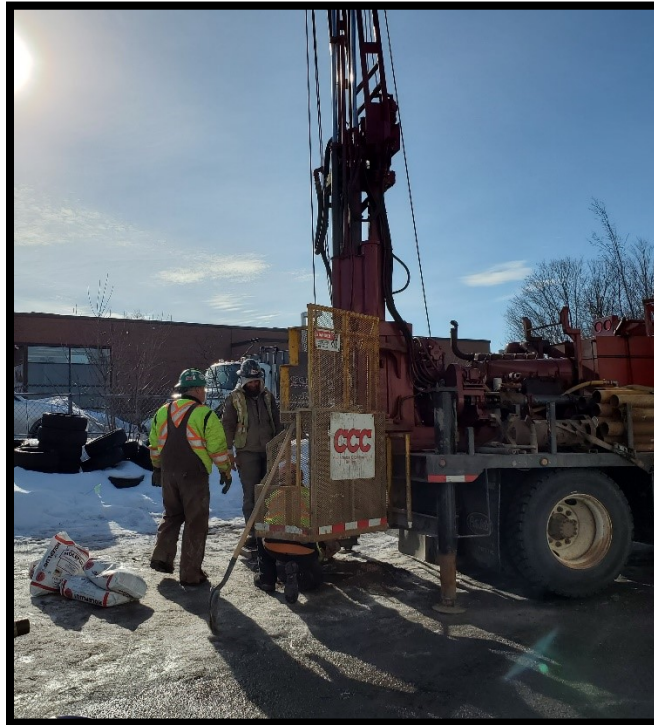
Photograph 7: View of the advancement of BH21-1, facing southeast (March 10, 2021)
