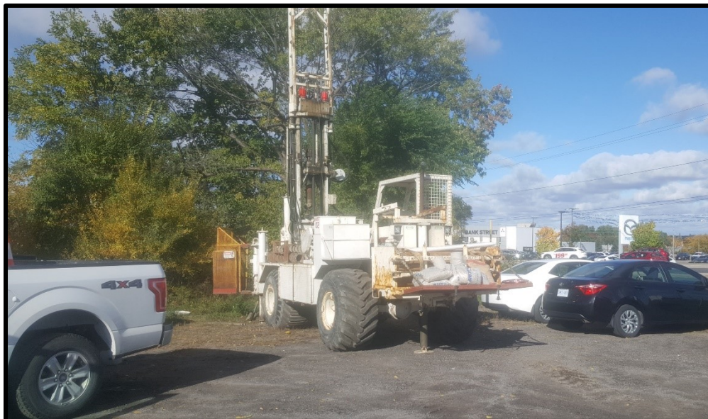
Photograph 6: View of the advancement of BHMW18-3, facing northwest (October 12, 2018)
