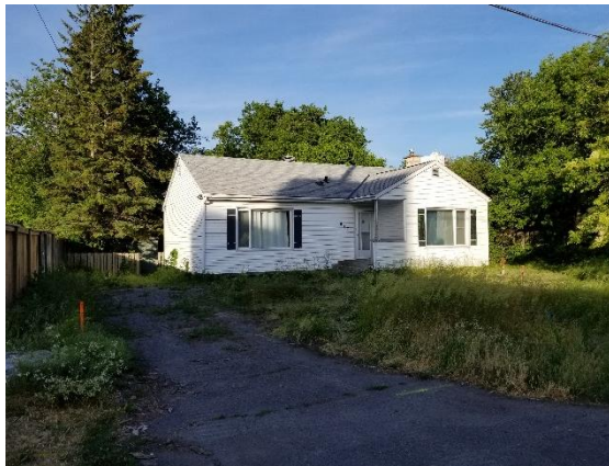
Figure 2-2: Existing one-storey single-detached dwelling
