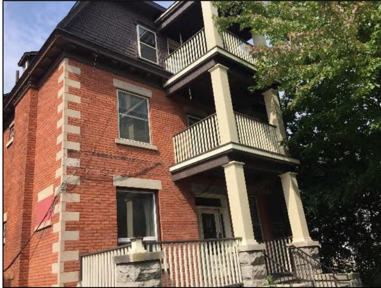
Photo 1 – Site Building (northeast elevation).
