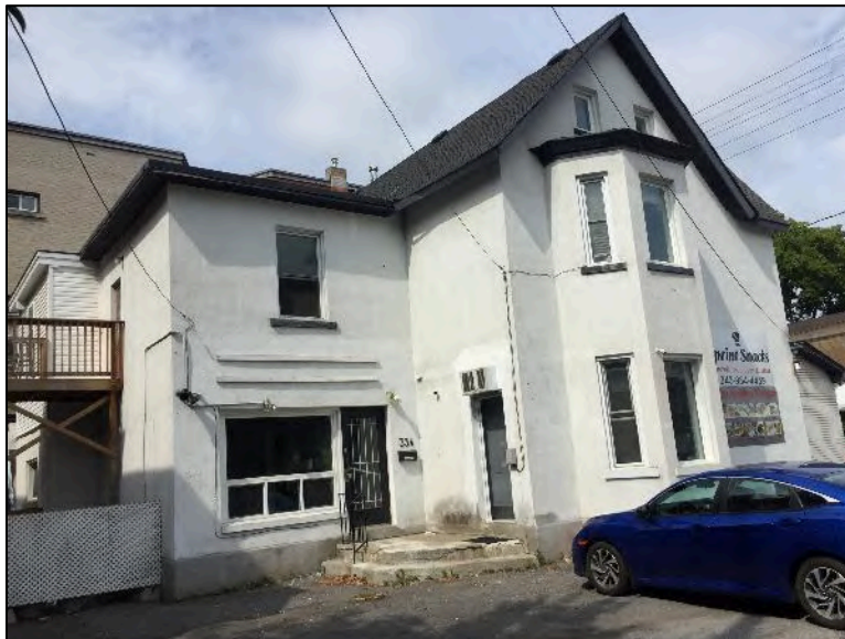
Photo 6 – Property located northwest of the Phase One Property.
