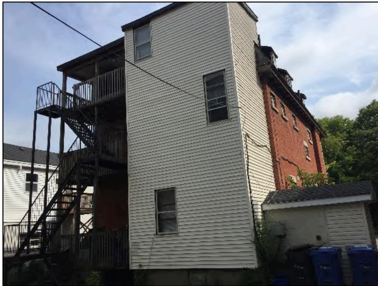
Photo 4 – Site Building (southwest elevation).
