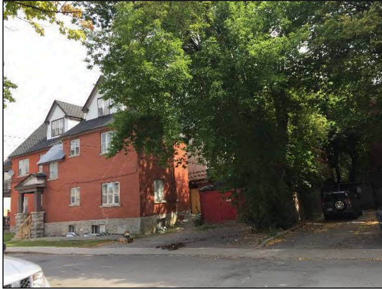
Photo 5 – Property located northeast of the Phase One Property.
