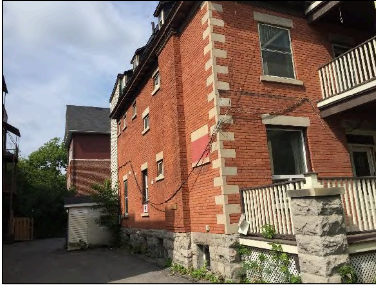
Photo 3 – Site Building (southeast elevation).
