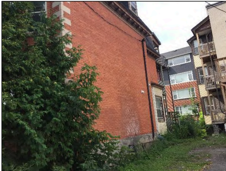
Photo 2 – Site Building (northwest elevation).
