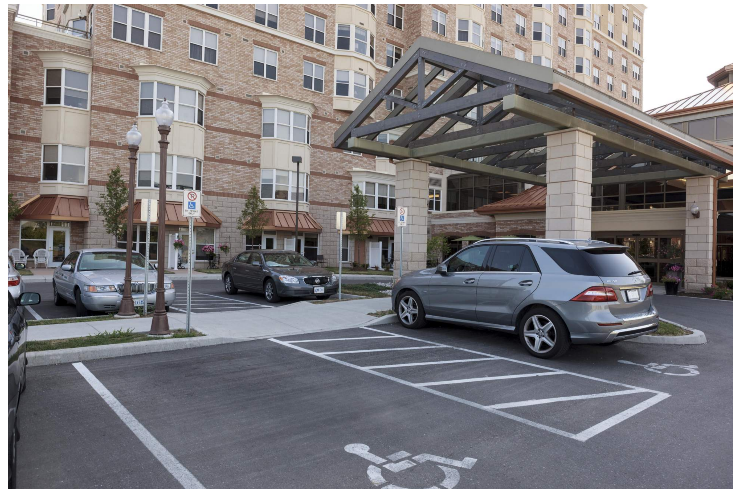
SUITE ENTRANCES AT GRADE
