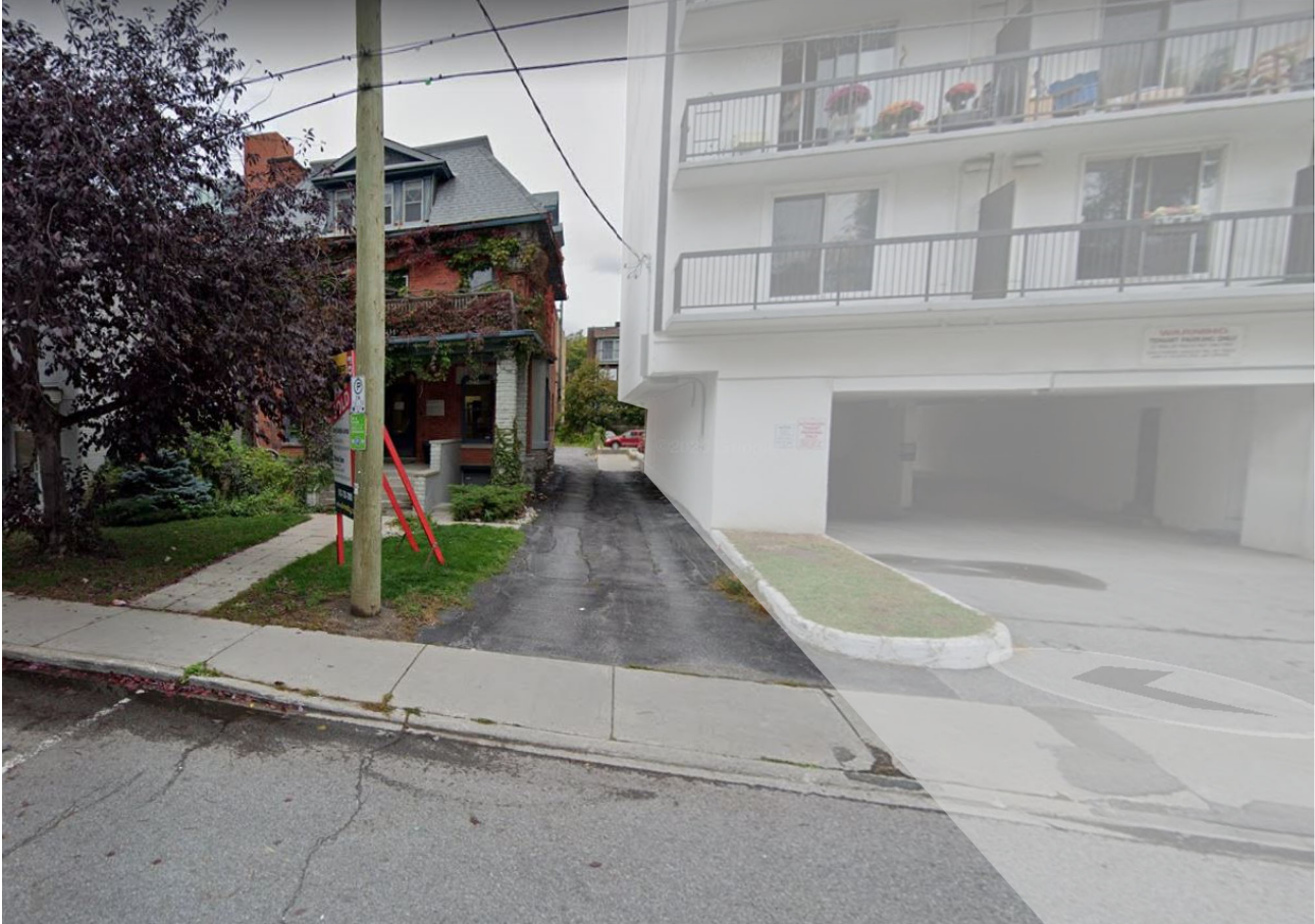
Figure 2: Existing building located on the subject property
