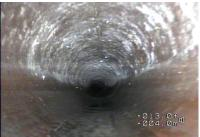
Figure#6: A view to the light encrustation at 9.2 meters from the top of TOILET FLANGE (TF1).
