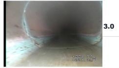
Figure#5: A view to the 10% water level and silt under water at 6.2 meters from the top of CATCH BASIN 1 (CB1).
