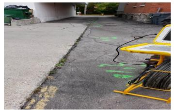
**Figure#4** A view to line STM1orientation and depth in the alley. 3 feet and 11 inches.
