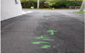
**Figure#7** A view to the line STM2 in Argyle Street. It is 7 feet in the middle then drops to 9.5 to 10 feet the main line.
