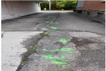
**Figure#2** A view to line STM1orientation and depth in the alley. 2 feet and 10 inches deep.
