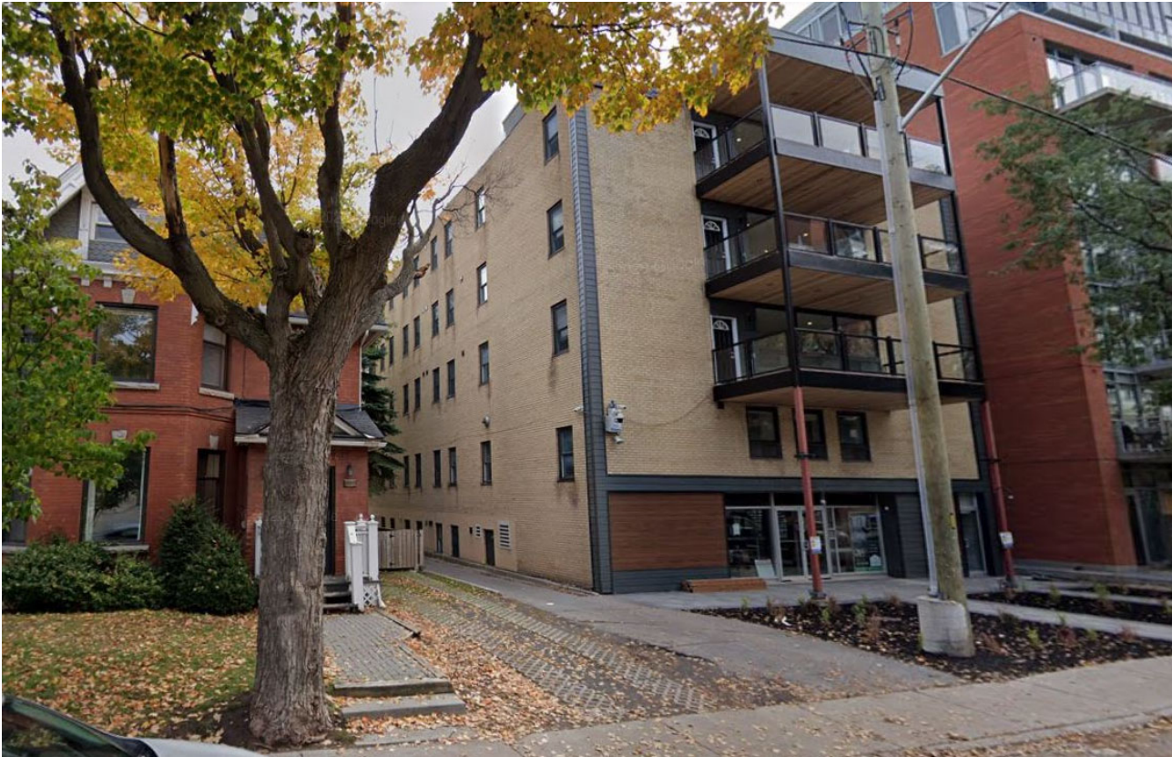
Figure 2: Existing building located on the subject property
