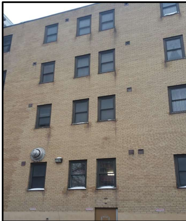
Photograph 2: Rear view of subject building looking north.
