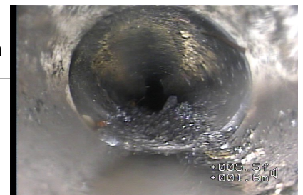
Figure#6: A view to the material change to No corrode and sand/silt at 1.8 meters from the top of CATCH BASIN 1
