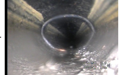
Figure#10: A view to the 10% water level at 6 meters from the top of CATCH BASIN 1 (CB1).
