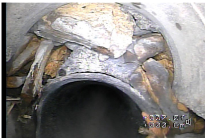
Figure#5: A view to the Oval joint due to deformation at 4.0 meters from the top of CATCH BASIN 2 (CB2).
