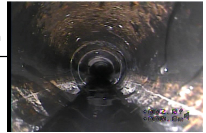
Figure#4: A view to the wye connection to the line CITY MAIN LINE at 3.4 meters from the top of TOILET FLANGE
