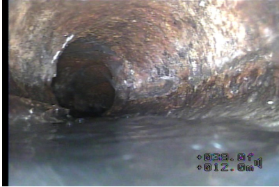
Figure#15: A view to the 10% water level at 15.6 meters from the top of TOILET FLANGE (TF1).
