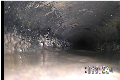
Figure#15: A view to the material change to No corrode at 15.4 meters from the top of CATCH BASIN 1 (CB1).
