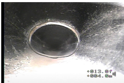
Figure#5: A view to the Oval joint due to deformation at 4.0 meters from the top of CATCH BASIN 2 (CB2).
