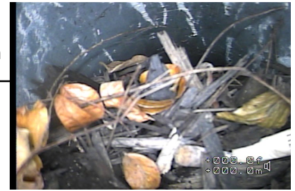
Figure#4: A view to the 100 mm TEE connection and left deviation at 0.8 meters from the top CATCH BASIN 3
