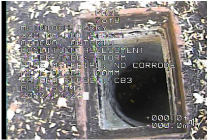
Figure#3: A view to the line deviation downwards and medium offset joint at 0.2 meters from the top of (CB3).
