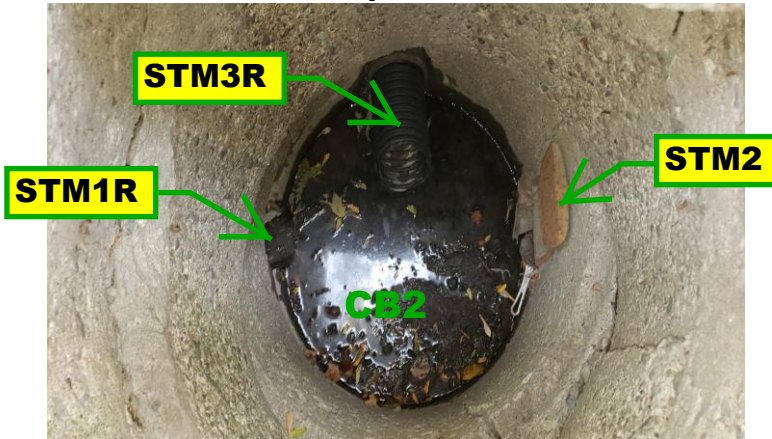
Figure#7 A view to the pipe STM2 orientation. It pics up line STM3.
