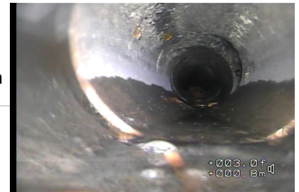
Figure#6: A view to the material change to No corrode and sand/silt at 1.8 meters from the top of CATCH BASIN 1
