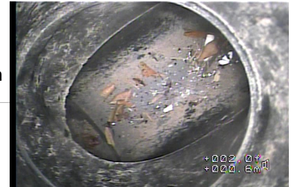
Figure#4: A view to the 100 mm TEE connection and left deviation at 0.8 meters from the top CATCH BASIN 3
