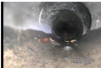
Figure#5: A view to the 100mm 3 o'clock connection at 1.2 meters from the top CATCH BASIN 1 (CB1).
