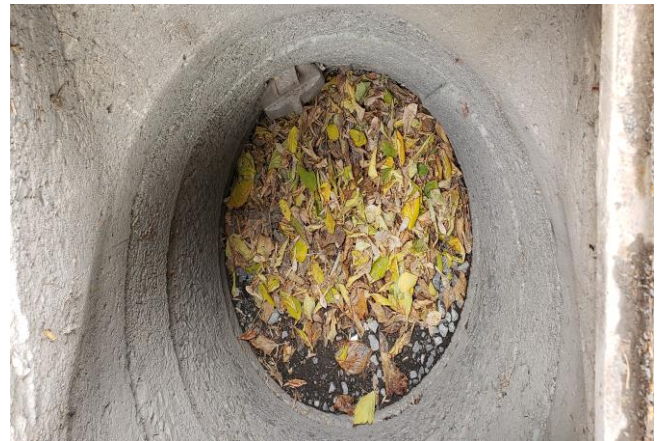
Figure#4 A view to catch basin CB2 in the driveway
