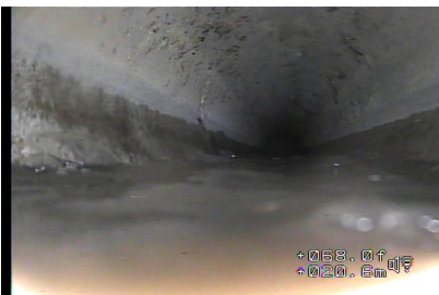
Figure#17: A view to the 20% water level at 20.8 meters from the top of CATCH BASIN 1 (CB1).
