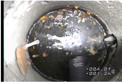
Figure#3: A view to the 10% of the pipe's surface area lost due to the deformed pipe at 0.4 meters from the top of CATCH BASIN 1 (CB1).
