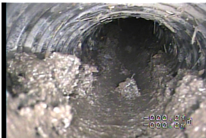
Figure#3: A view to the 10 % Debris Silt and sand at 0.4 meters from the top of TEE.
