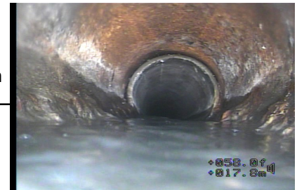
Figure#18: A view to the material change to PVC at 22.2 meters from the top of TOILET FLANGE (TF1).
