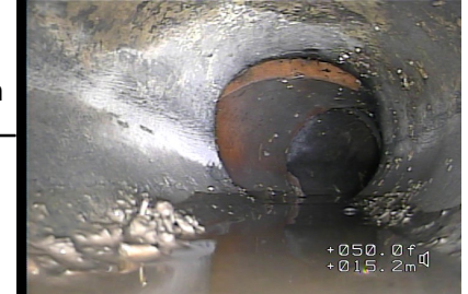
Figure#16: A view to the 20% Debris at 15.8 meters from the top of CATCH BASIN 1 (CB1).
