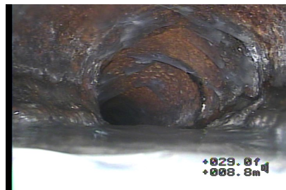
Figure#11: A view to the 20% water level and 12 o'clock connection at 11.6 meters from the top of TOILET FLANGE (TF1).
