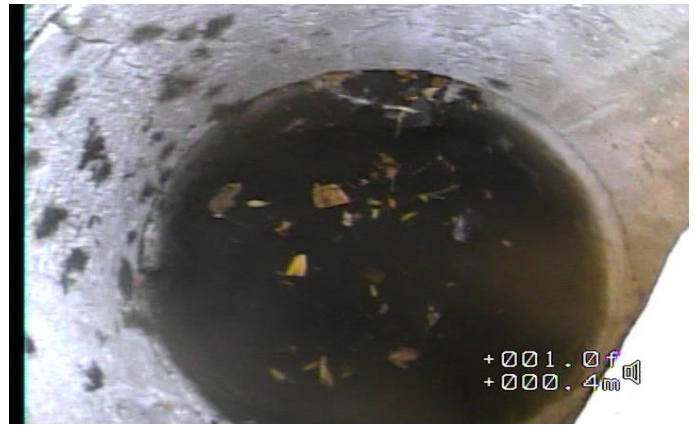
Figure#20 The Water main feed is 38.1 mm diameter.
