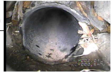
Figure#4: A view to the 10% deformed pipe at 1.8 meters from the top of CATCH BASIN 2 (CB2).
