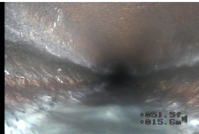
Figure#17: A view to the 3 o'clock connection intruding about 0.25 mm at 21.2 meters from the top of (TF1).
