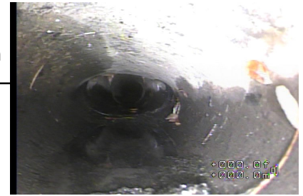
Figure#4: A view to the material change to PVC at 1.2 meters from the top of CATCH BASIN 1 (CB1).
