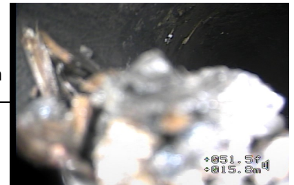
Figure#18: A view to the material change to PVC and right deviation at 22.2 meters from the top of CATCH BASIN 1 (CB1).
