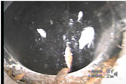
Figure#3: A view to the line deviation downwards and medium offset joint at 0.2 meters from the top of (CB3).
