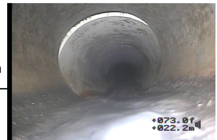
Figure#18: A view to the material change to PVC at 22.2 meters from the top of TOILET FLANGE (TF1).
