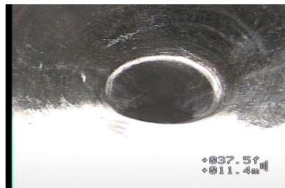
Figure#11: A view to the 0% water level and deformed pipe at 13.4 meters from the top of CATCH BASIN 2 (CB2).
