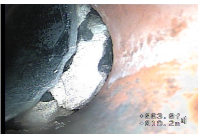
Figure#17: A view to the material change to No Corrode and offset joint at 19.2 meters from the top of CATCH
