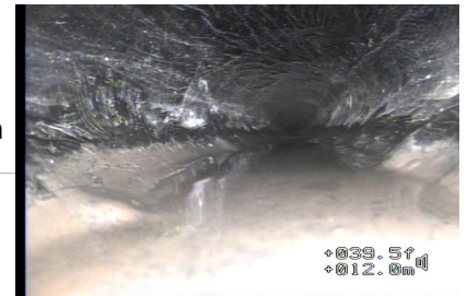
Figure#12: A view to the 10% deformed pipe at 14.0 meters from the top of CATCH BASIN 2 (CB2).
