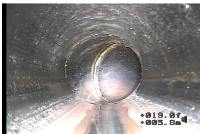
Figure#5: A view to the right line deviation at 5.8 meters from the top of TOILET FLANGE (TF1).
