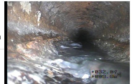
Figure#12: A view to the 150mm 12 o'clock connection at 11.8 meters from the top TOILET FLANGE (TF1).
