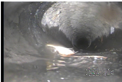
Figure#5: A view to the 100mm 3 o'clock connection at 1.2 meters from the top CATCH BASIN 1 (CB1).
