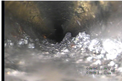
Figure#9: A view to the 10 % Debris gravel at 5.0 meters from the top of CATCH BASIN 1 (CB1).
