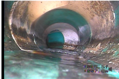
Figure#9: A view to the material change to cast iron at 9 meters from the top of TOILET FLANGE (TF1).
