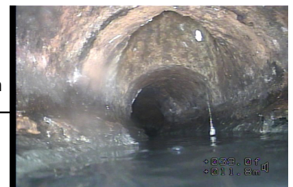
Figure#12: A view to the 150mm 12 o'clock connection at 11.8 meters from the top TOILET FLANGE (TF1).
