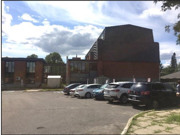
Figure 2-5: Parking area at rear of St. Thomas the Apostle Anglican Church looking west
