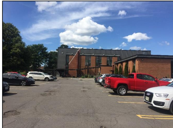
Figure 2-4: Parking area south of St. Thomas the Apostle Anglican Church looking north
