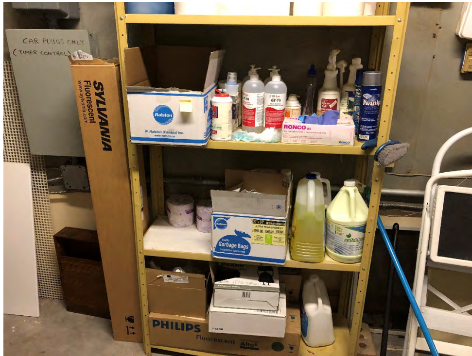
Photo 21 Photo showing the cleaning chemicals stored in the electrical room of Ellwood House Seniors' Residence
