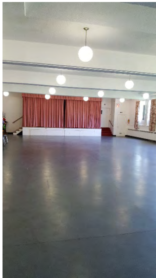
Photo 8 - View of the interior of the basement level of the Church building.
