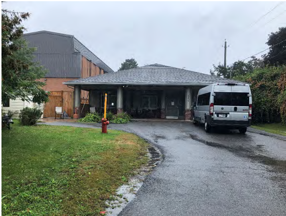
Photo 7 Photo showing the Recreational Services building, facing west
