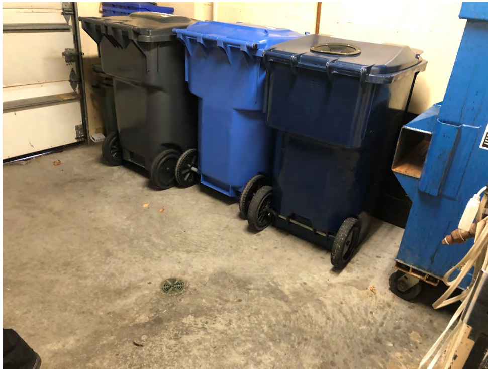
Photo 23 View of the garbage room at Ellwood House Seniors' Residence
