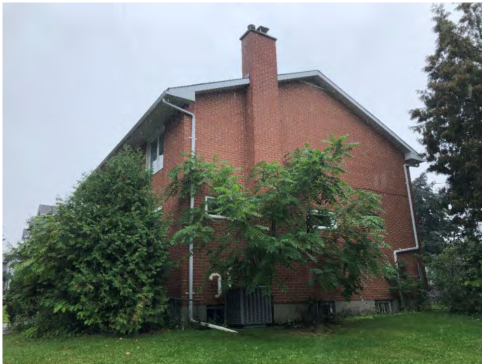
Photo 6 Photo showing the private residence, facing south
