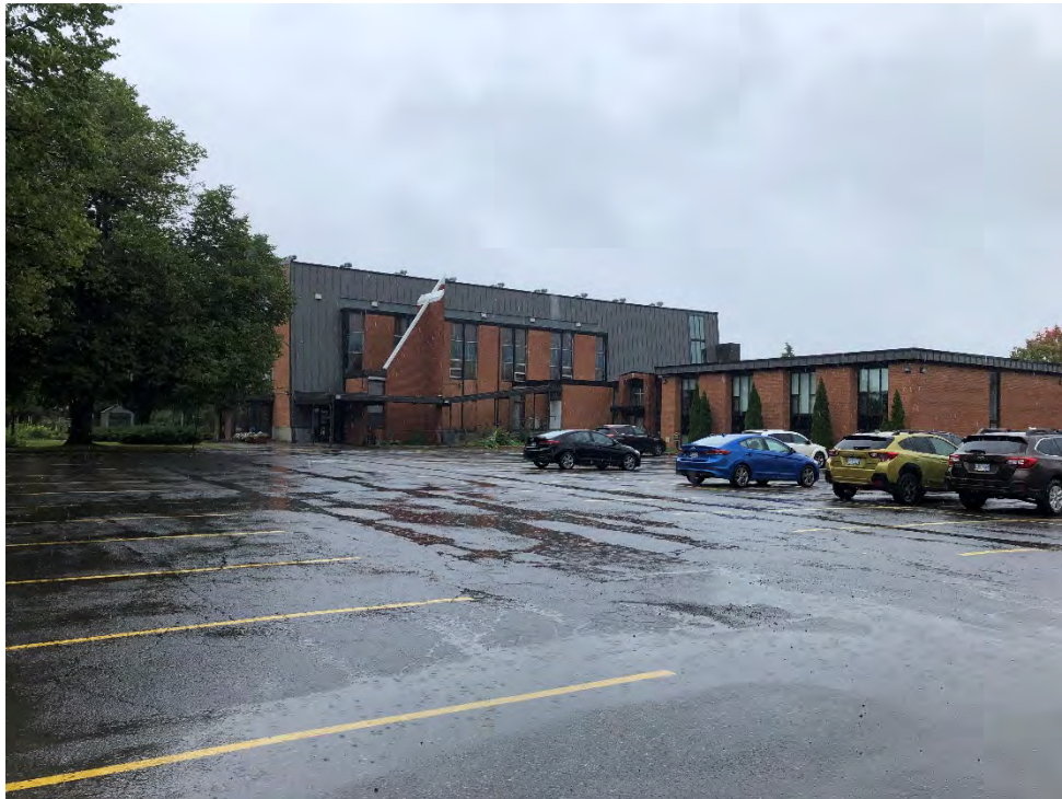
Photo 2 View of the church and asphalt parking area, facing northeast
