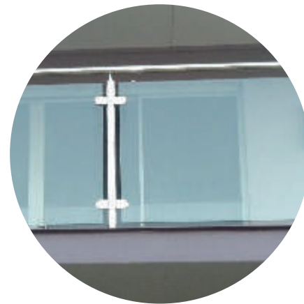
7. BALCONY METAL SIDING
