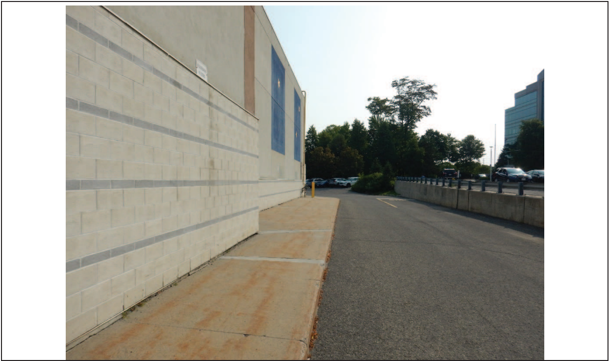
Photo 15: View of the southern property boundary and neighbouring properties (facing east)
