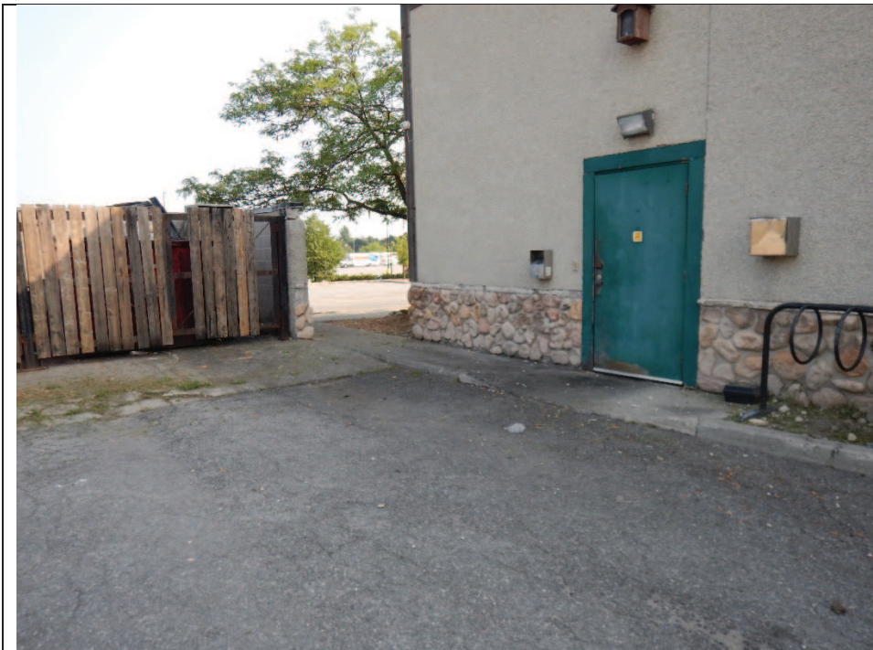
Photo 21: View of the northwestern corner of the Montana's and garbage bin (facing northeast)
