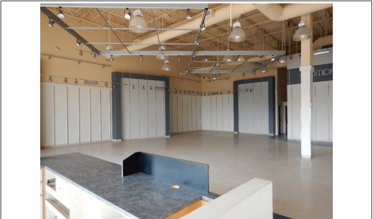
Photo 6: Interior of the vacant portion of the commercial retail space on the Phase One Property (facing west)
