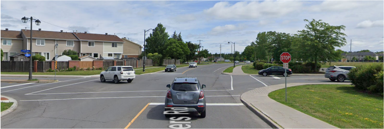
Figure 3: Looking East Along Watters Road from the Subject Property West Access
