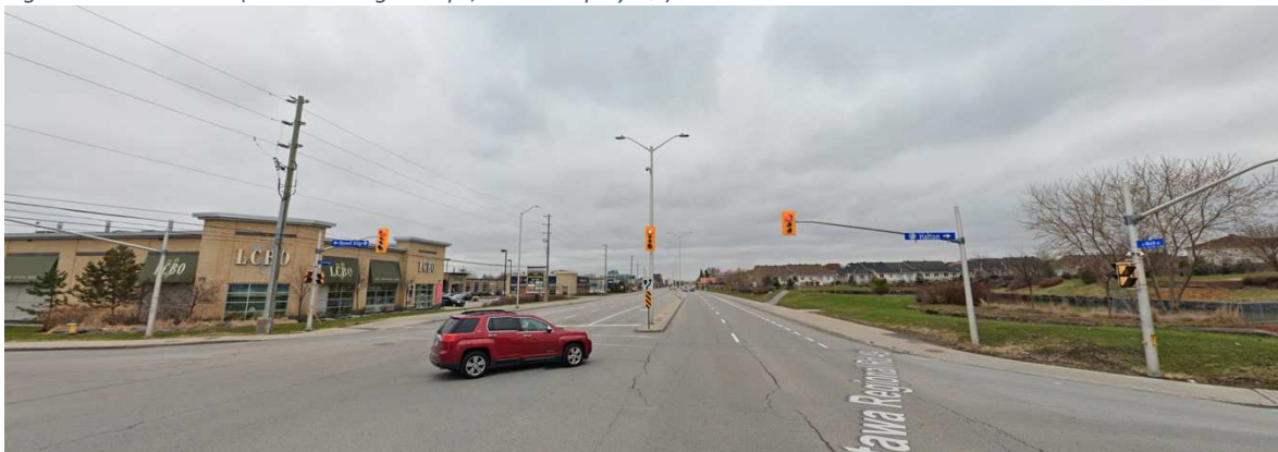
Figure 7: View looking south on March Road at Halton Terrace intersection. (Source: Google Streetview).
