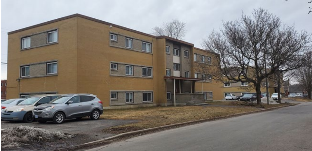
Figure 2-9 Three-storey apartment buildings south of the site along Borthwick Ave
