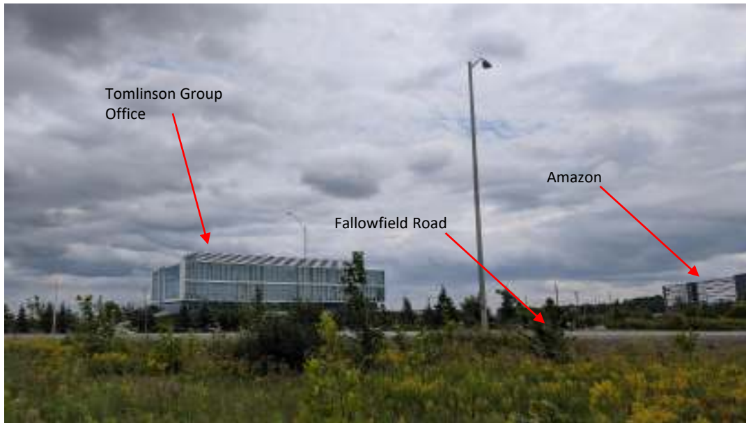
Photograph 19: New office construction south beyond Fallowfield Rd.
