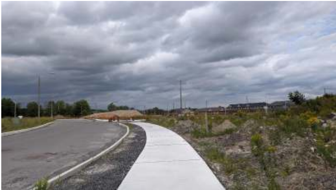
Photograph 21: Beyond east side Hampton Inn & Suites along Lusk St. Undeveloped land with stockpiles of fill. (Photo facing northeast on Lusk St.)
