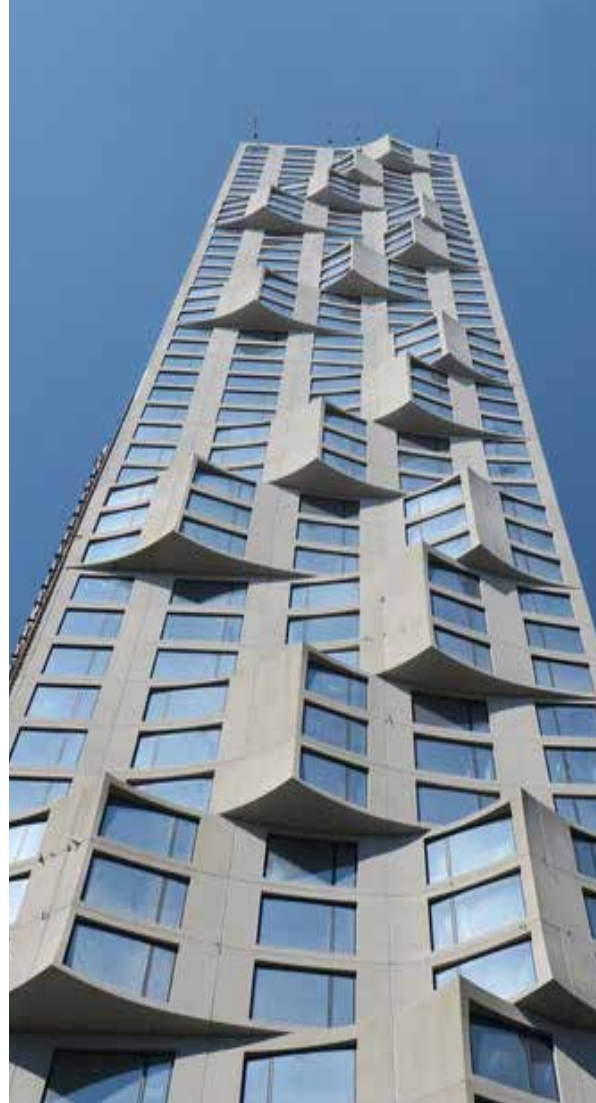
Pattern development on the tower
