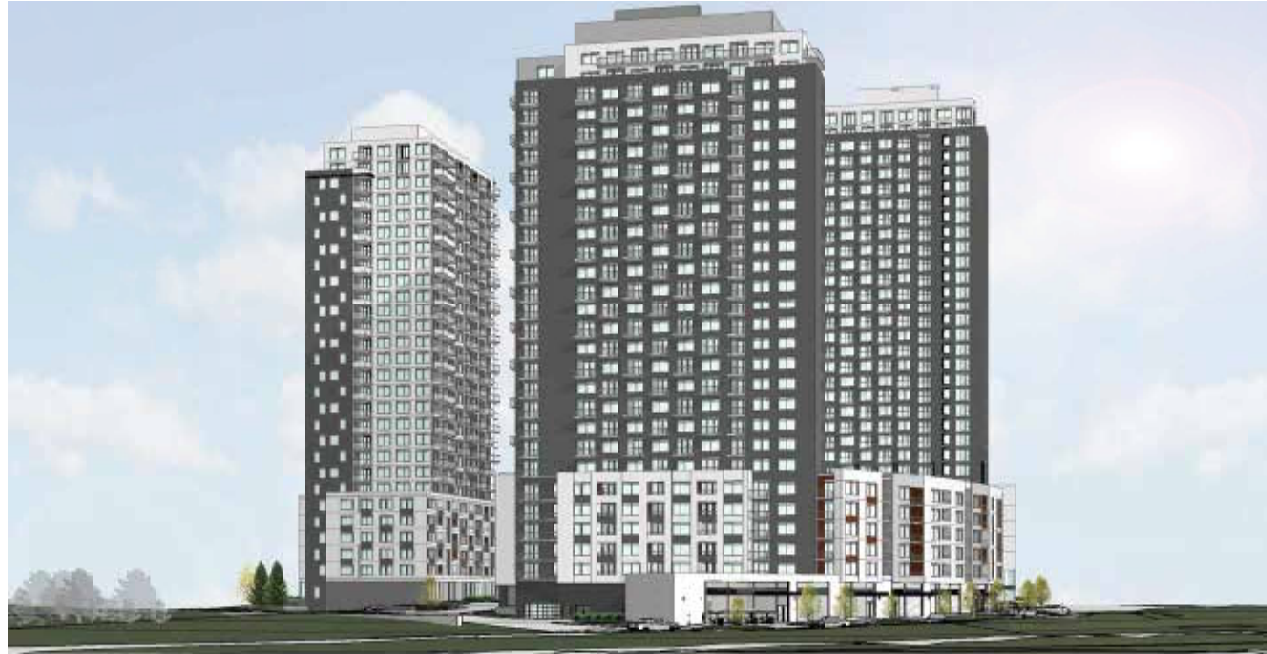
VIEW LOOKING EAST
