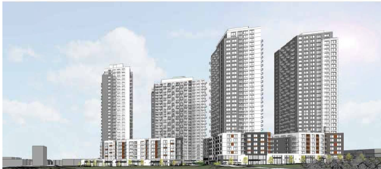
VIEW LOOKING NORTH
