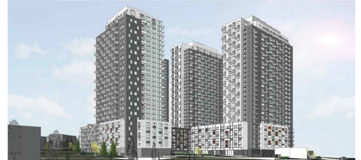
VIEW LOOKING SOUTH EAST
