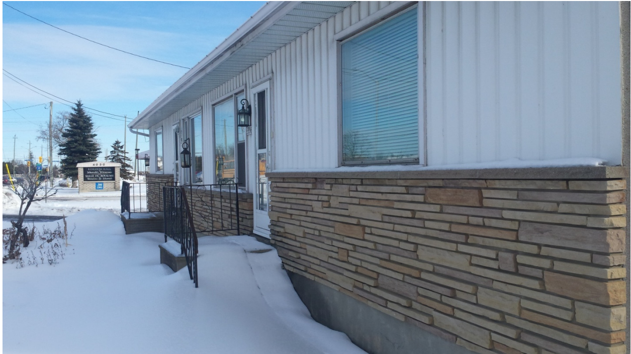
Photograph 1: Front view of the subject building, looking east.
