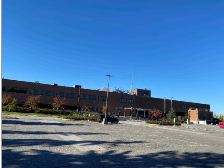
Photo 9 – Electronic and computer equipment manufacturer located adjacent to the southwest elevation of the Phase One Property (PCA #1).
