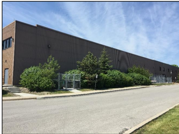
Figure 2-9: North face of existing building at 415 Legget, looking south
