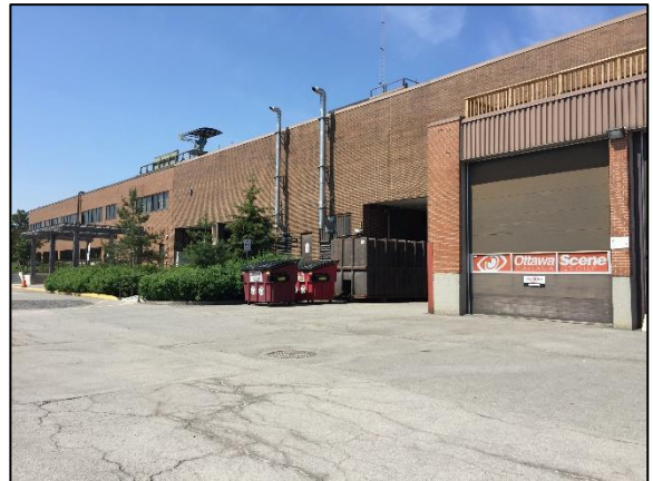
Figure 2-8: East face of existing building at 415 Legget, looking west
