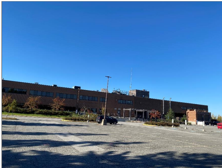
Photo 8 – Property located southwest of the Phase One Property.
