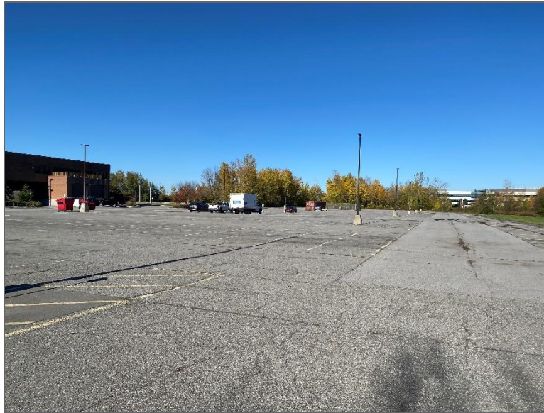
Photo 1 – View from the southeast portion of the Phase One Property, looking northwest.
